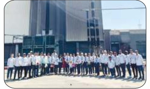
HVDC Substation, Padghe
